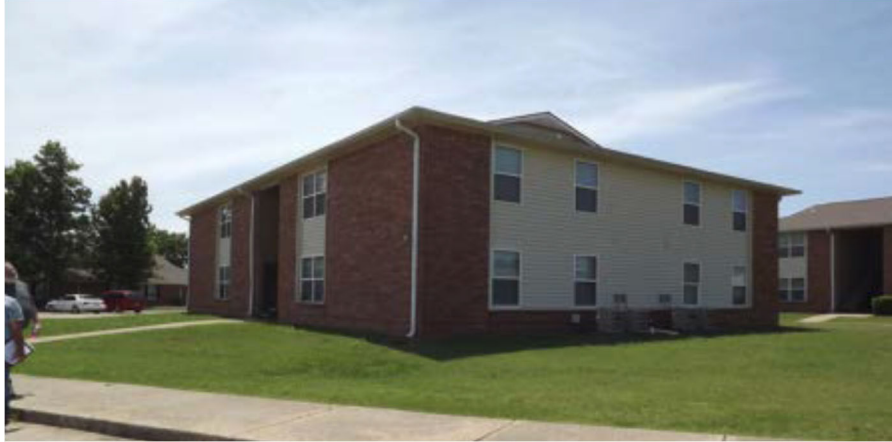
Skiatook (Prior to Rehabilitation)
