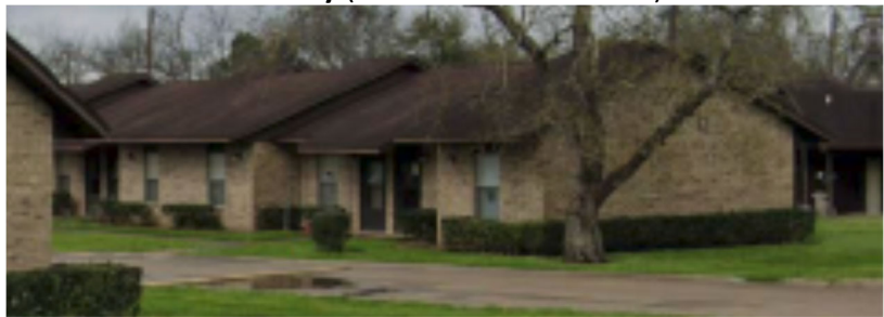
Sweeny (Prior to Rehabilitation)
