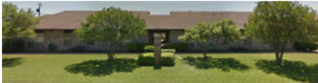
Pearsall (Prior to Rehabilitation)
