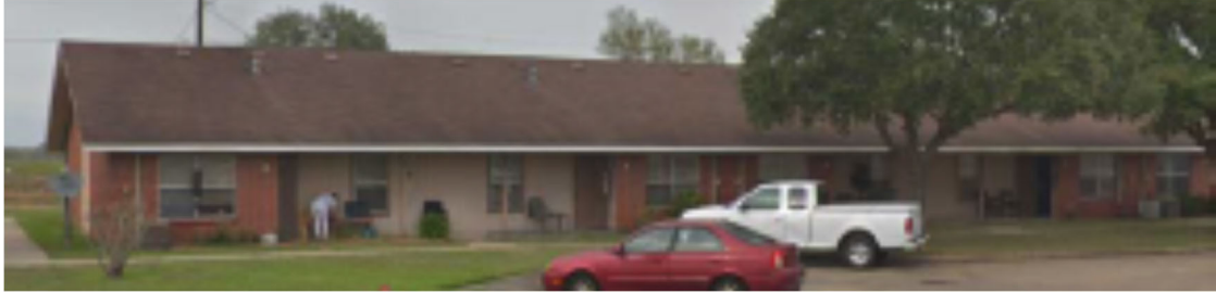
Hempstead (Prior to Rehabilitation)
