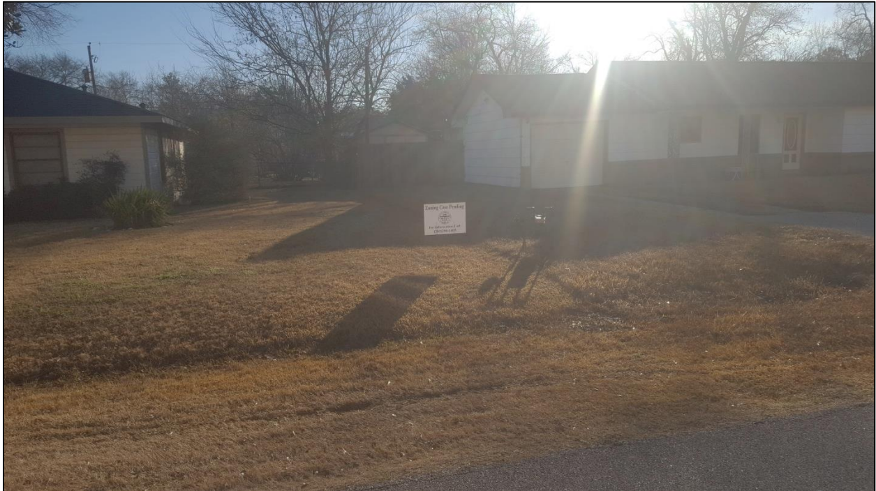
Subject site view from Raymond Street
