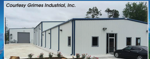
Grimes Industrial, Inc.'s new Corporate Office and Fabrication facility located at 929 E. Main St. in Tomball, TX
