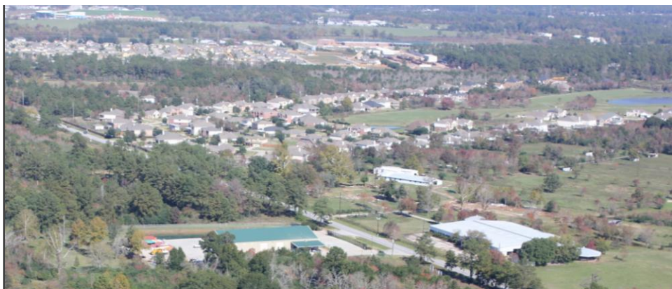
Figure 5: Hufsmith-Kohrville Road, single-family residences, and a former horse training facility.
