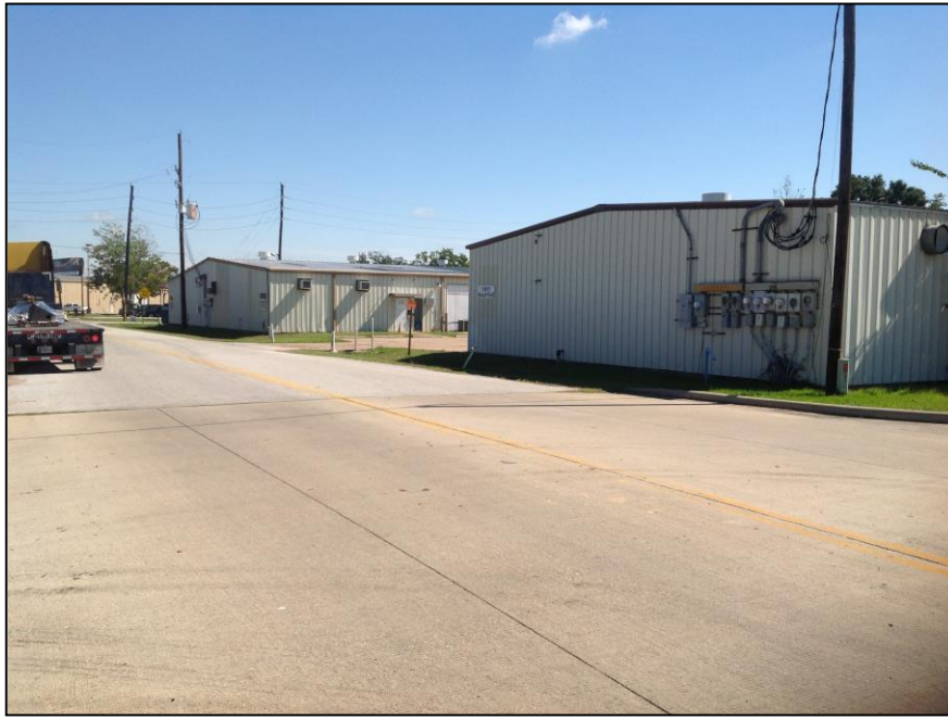
Figure 7: Office/warehouses to the west.
