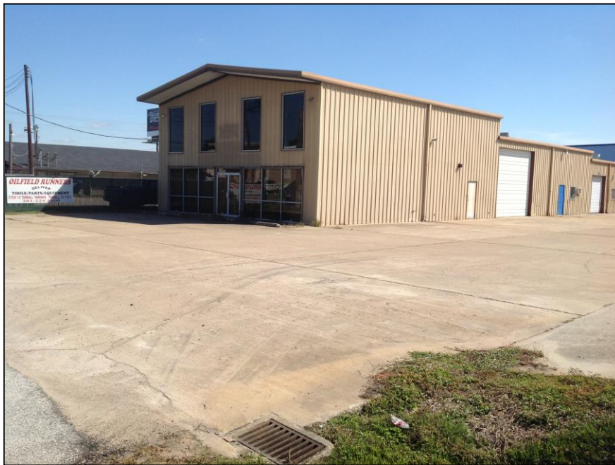
Figure 12: Office/warehouse to the east.
