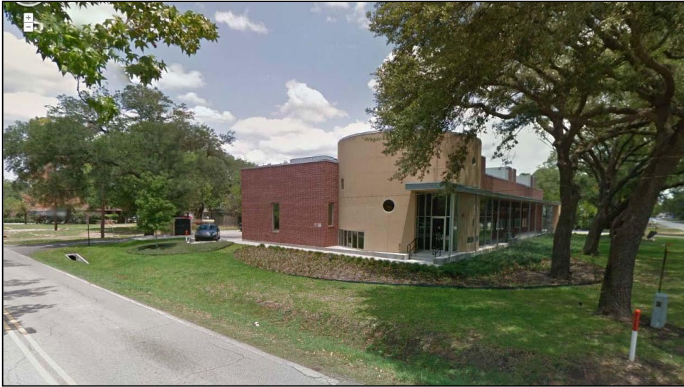
Figure 1: Subject site. Source: maps.google.com
