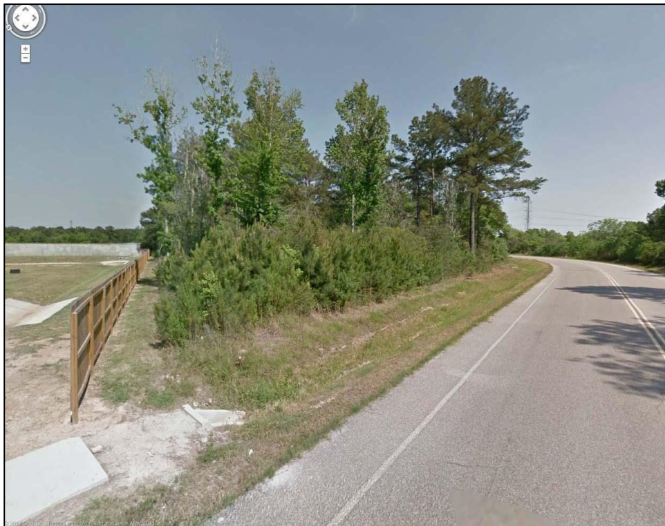
Figure 6: South of subject site.
