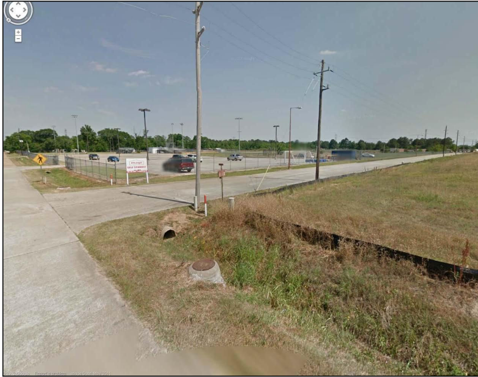
Figure 9: East of subject site.
