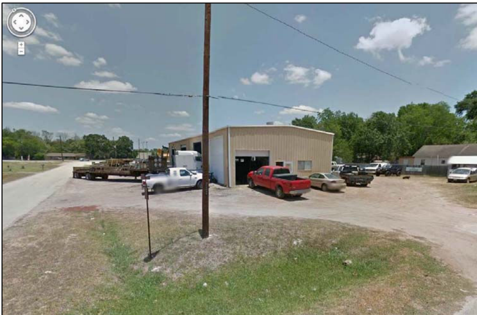
Figure 4: Auto service garage to the north. Source: maps.google.com
