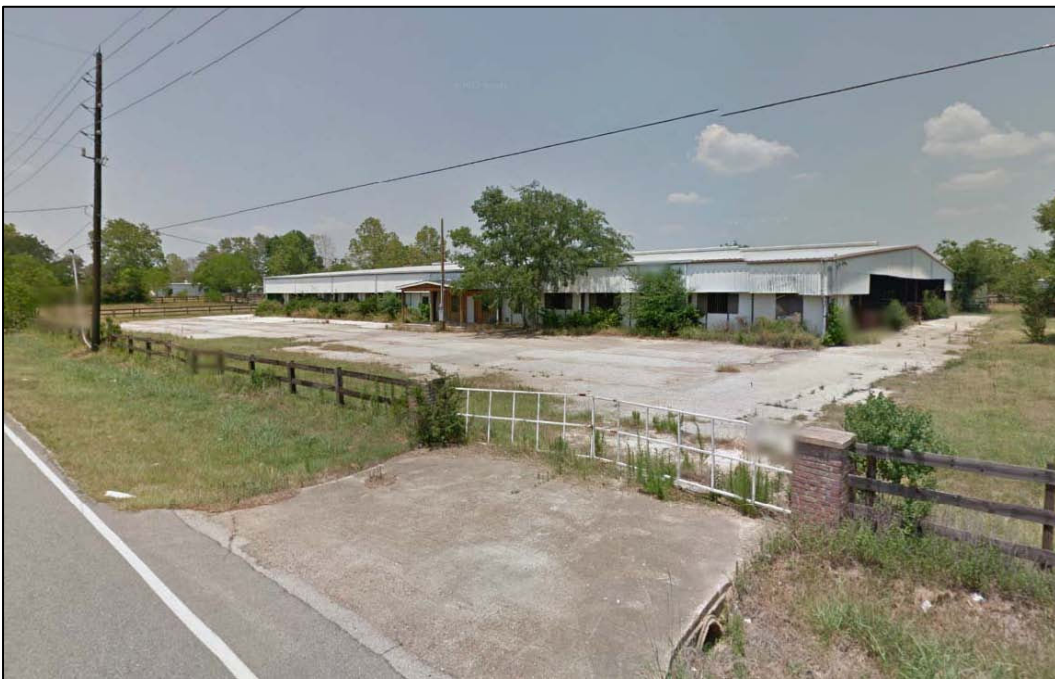
Figure 4: Former horse training facility to the east (maps.google.com).
