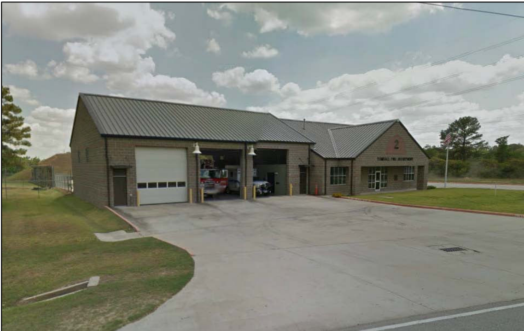
Figure 2: CoT fire station to the south. Source: maps.google.com
