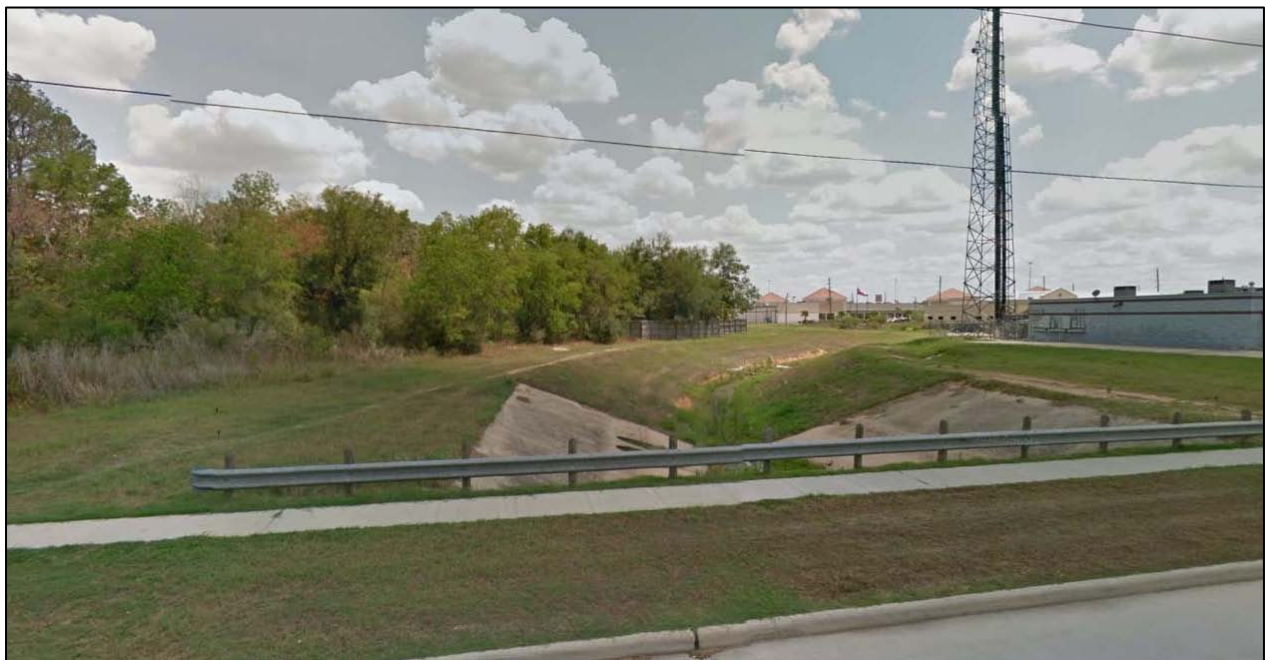
Figure 4: Drainage to the west. Source: maps.google.com
