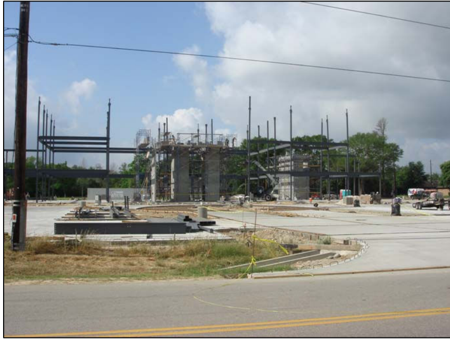
Figure 5: Medical office to the east. Source: maps.google.com
