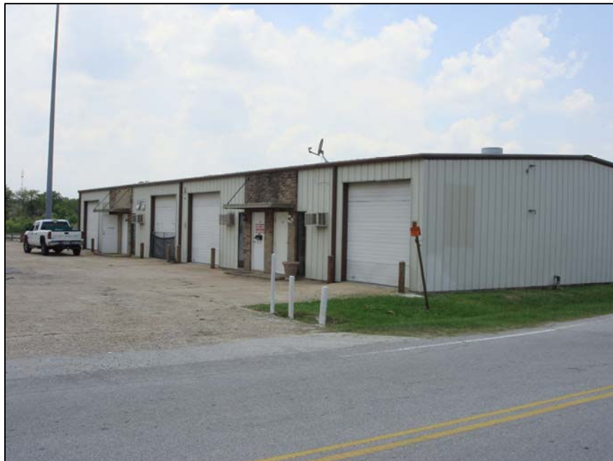
Figure 4: Warehouse building to the south.
