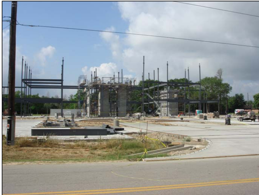
Figure 2: Medical office building being constructed to the north.
