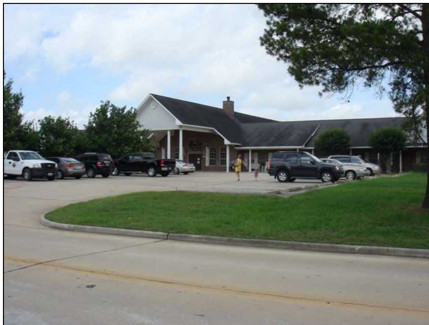
Figure 4: Assisted living facility to the west.
