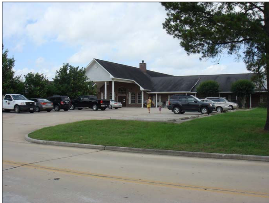
Figure 4: Assisted living facility to the west.
