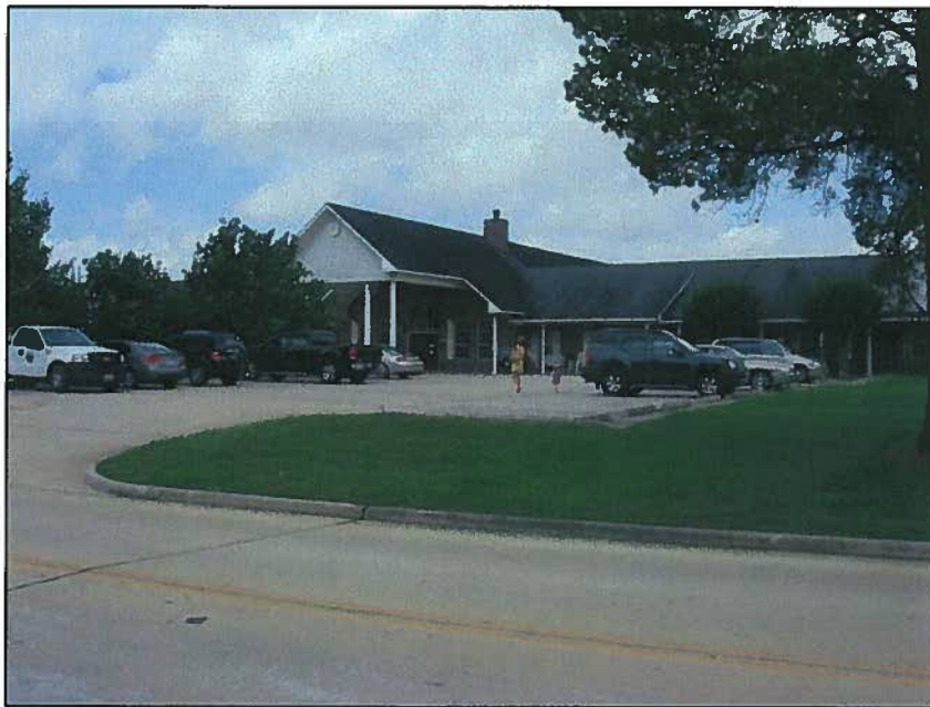
Figure 4: Assisted living facility to the west.
