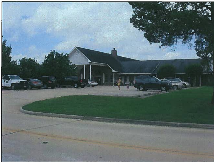
Figure 4: Assisted living facility to the west.
