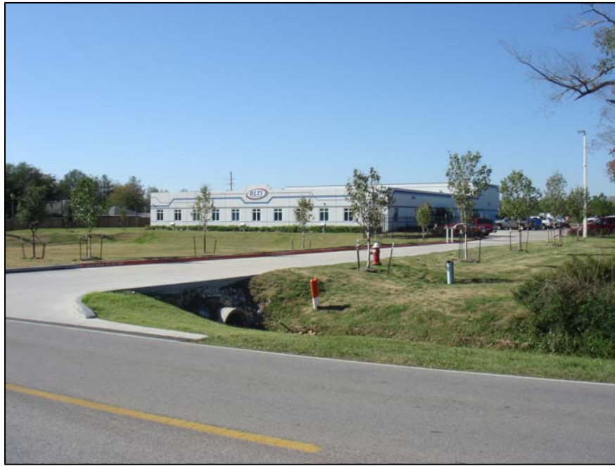
Figure 5: BL Technology to the south of subject site.
