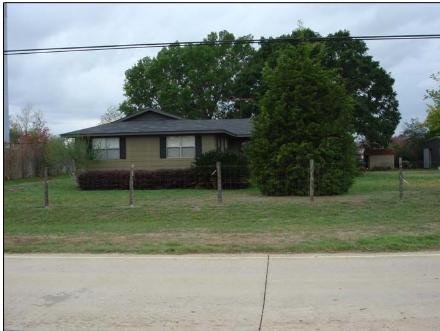
Figure 6: Residence to the northeast of subject site.
