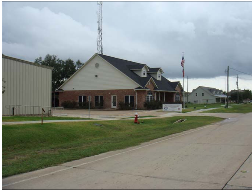
Figure 5: ESD station and office to the east of subject site.
