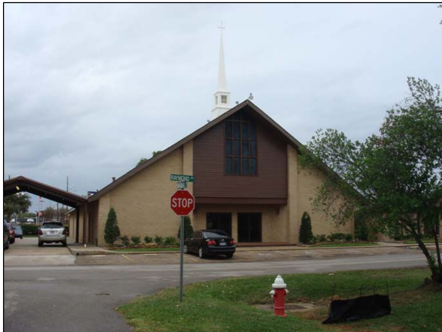
Figure 4: Church to the west of subject site.
