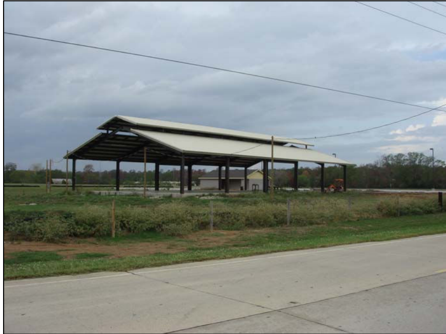
Figure 1: Westerly view of subject site.
