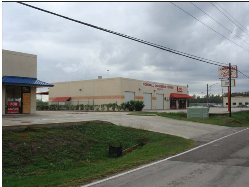
Figure 8: Commercial buildings to the northwest of subject site.
