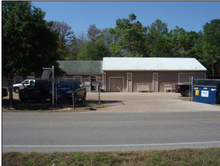
Figure 2: Northerly view of existing Abandoned Animal Rescue facility to the south of subject site.
