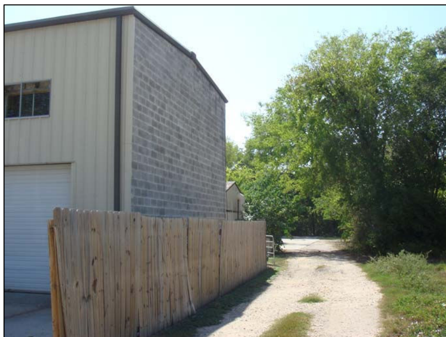
Figure 3: Northerly side of subject site.
