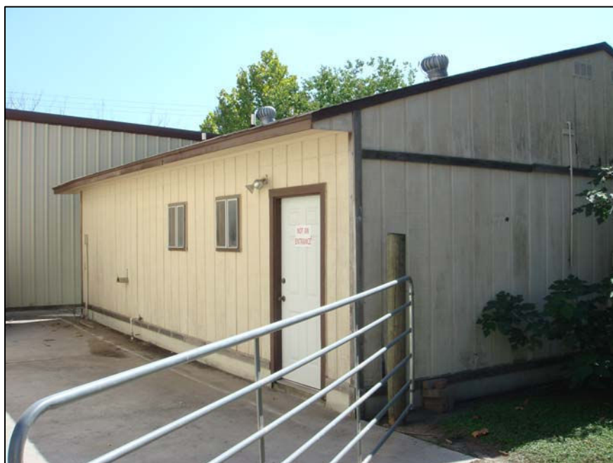
Figure 4: Northerly side of subject site.
