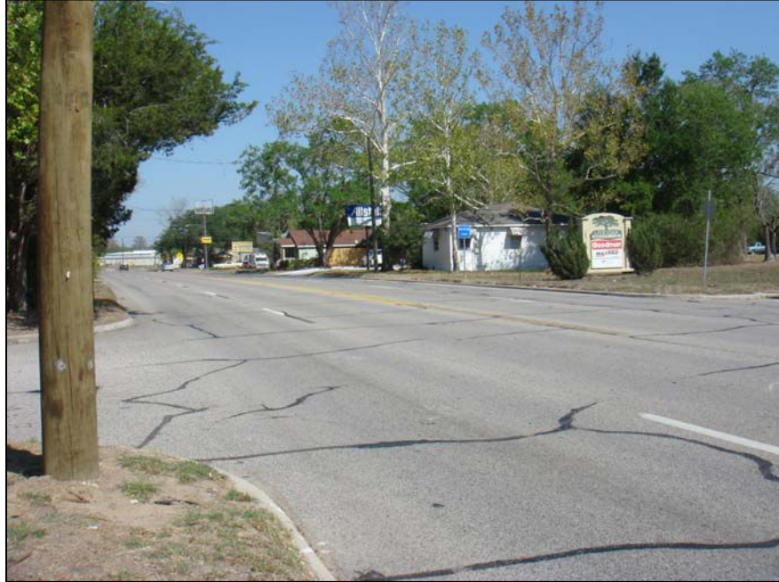
Figure 7: East of subject site.
