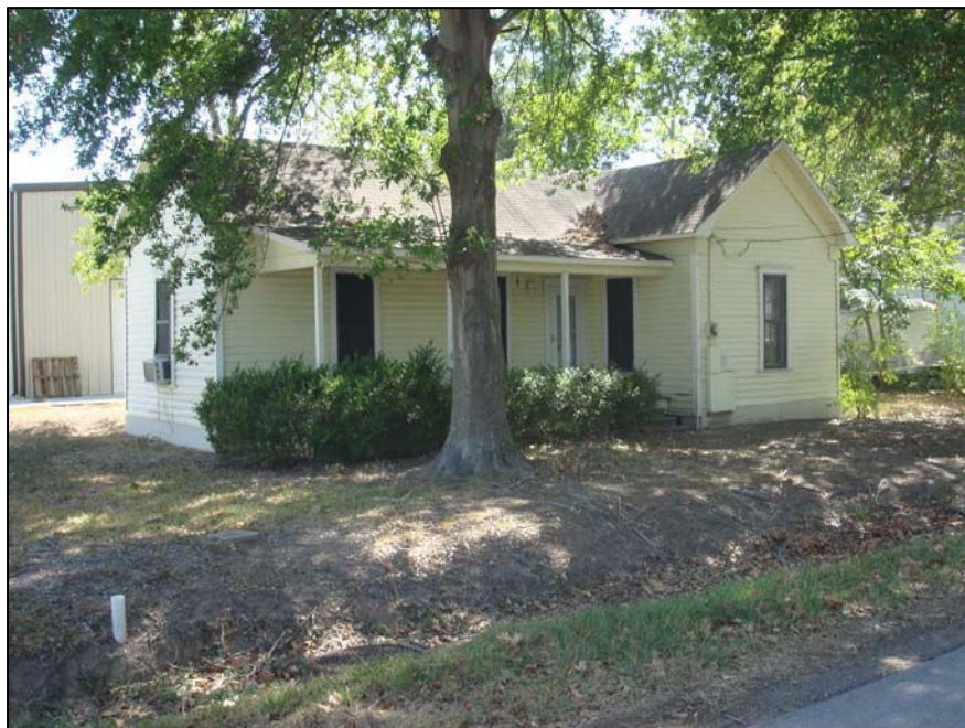
Figure 10: Residence to the north of subject site.
