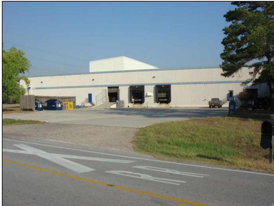
Figure 2: Houston Poly Bag to the west of subject site.
