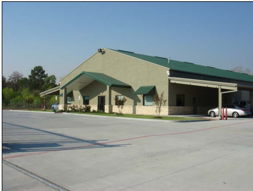
Figure 8: Creacom facility east of the subject site.
