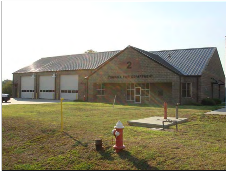
Figure 3: Tomball Fire Department Station #2 south of subject site.
