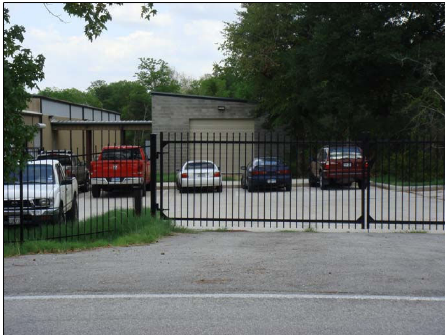
Figure 2: Easterly view of structure to be expanded.
