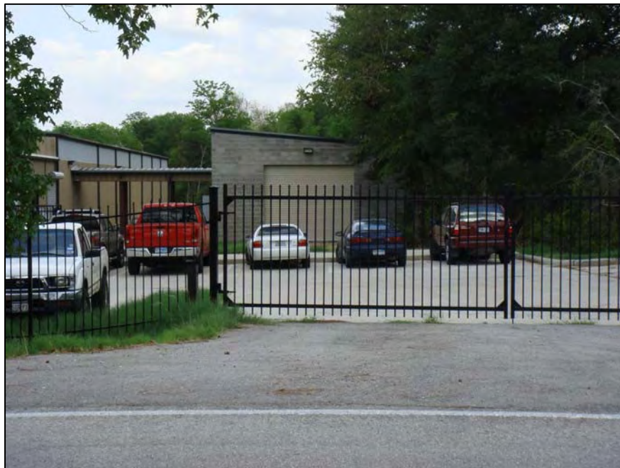
Figure 2: Easterly view of structure to be expanded.
