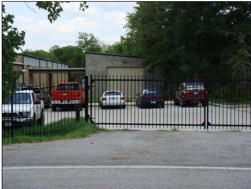
Figure 2: Easterly view of structure to be expanded.
