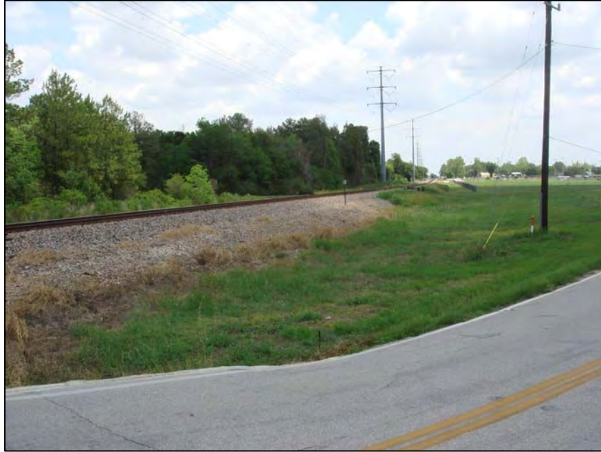
Figure 3: Southeasterly view. BNSF railway, City of Tomball property, and HCFCD drainage.
