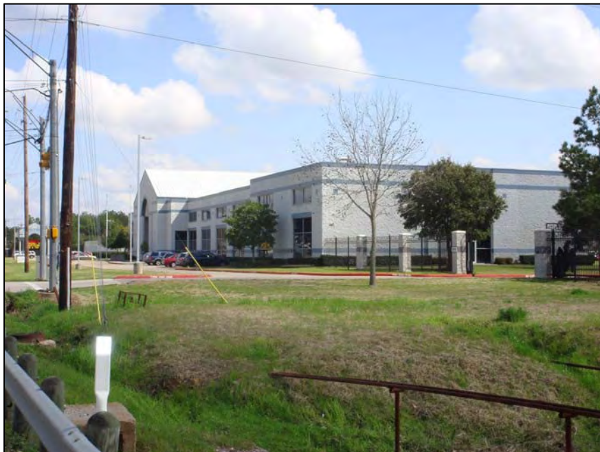
Figure 6: Harris County Flood Control District ditch and Concordia Lutheran School to the east of subject site.
