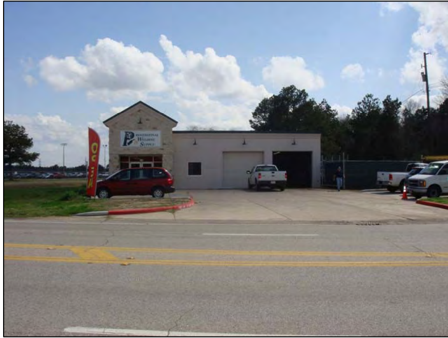
Figure 1: Southerly view of subject site.
