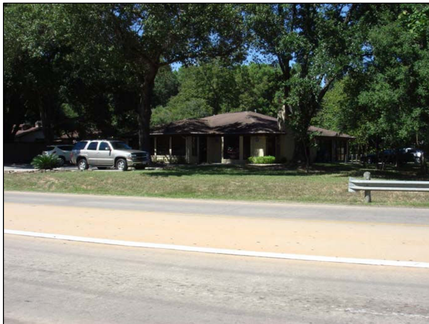
Figure 6: Insurance office to the south of subject site.
