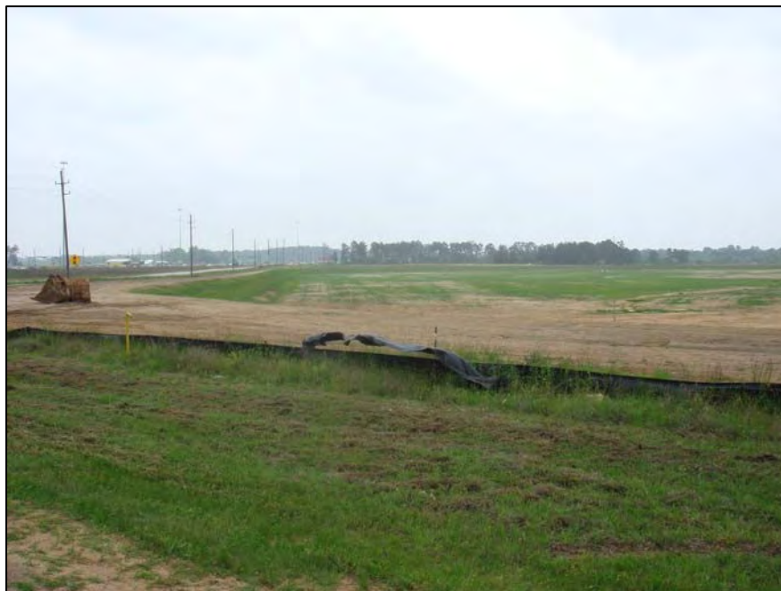
Figure 6: Harris County Flood Control District detention facility to the west of subject site.
