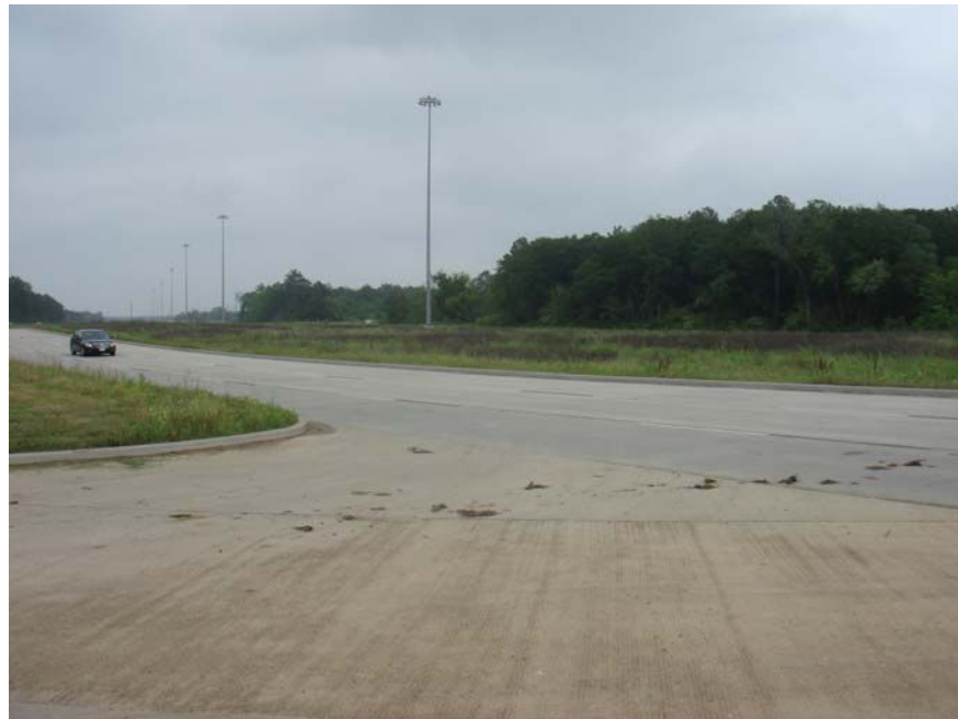
Figure 6: Northeasterly view of largely undeveloped portion of SH 249 Expressway. Subject site in center left of photo.
