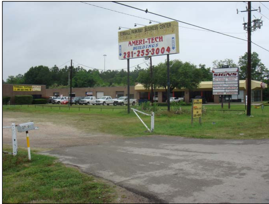
Figure 1: Northwesterly view of subject site.
