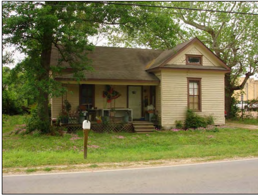
Figure 3: Existing single-family residence on southeast corner of subject site.
