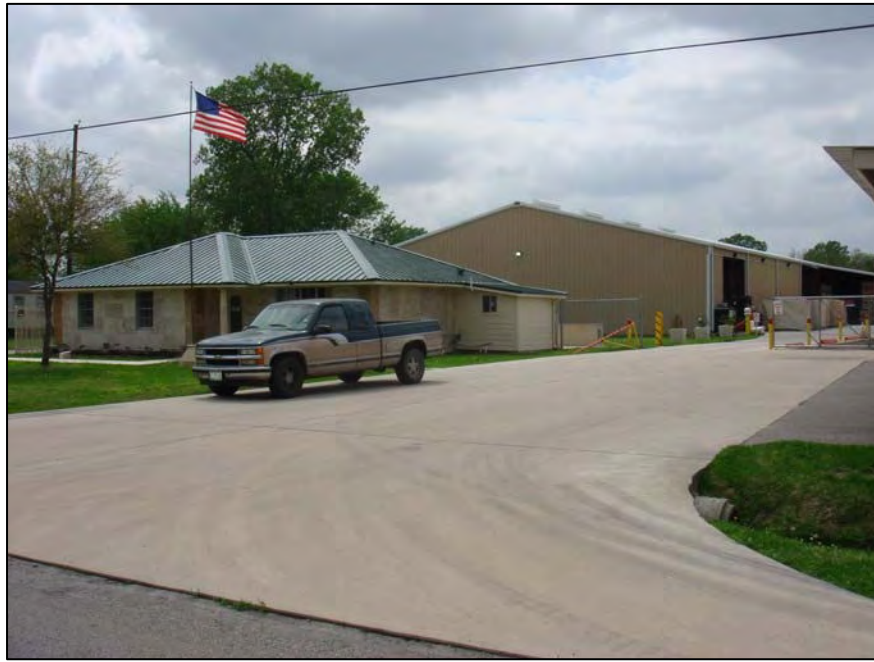
Figure 7: Rock processing facility to the north of subject site.
