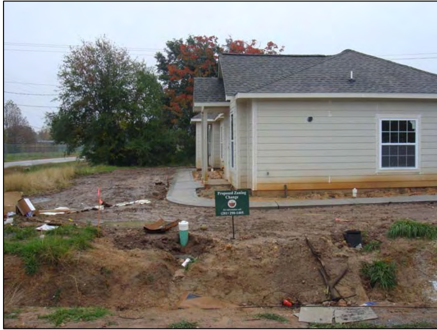
Figure 1: Easterly view of subject site.
