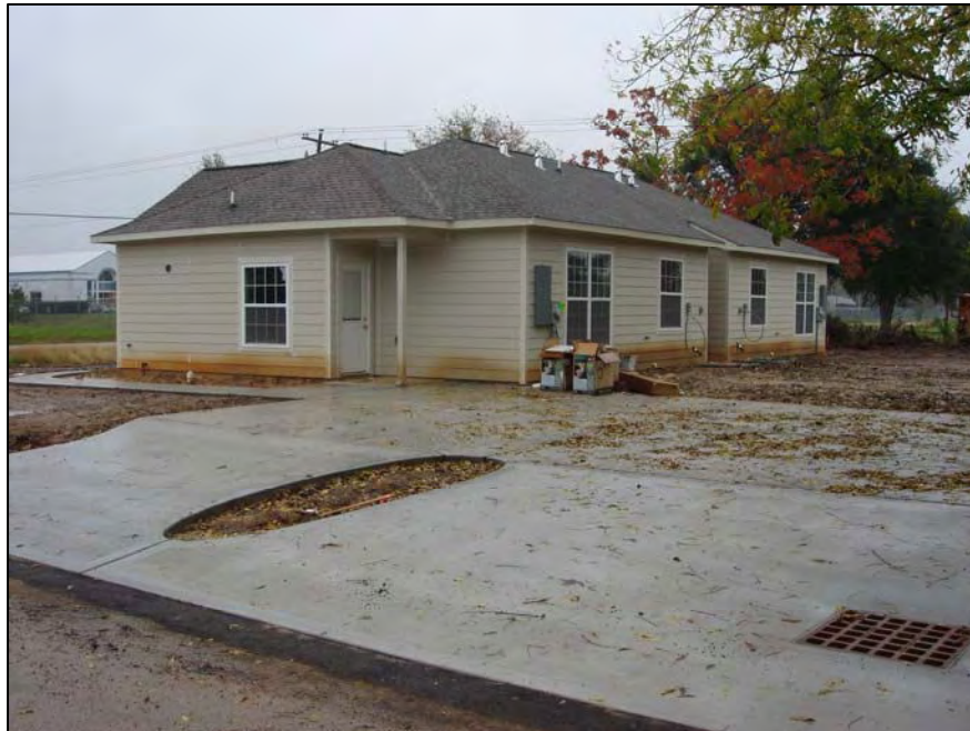
Figure 2: Northeasterly view of subject site.
