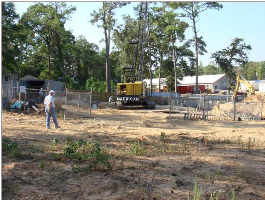
Figure 6: City of Tomball lift station being constructed on Lot 37 near subject site.
