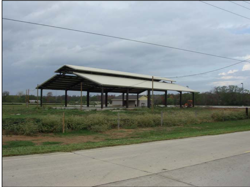
Figure 1: Westerly view of subject site.
