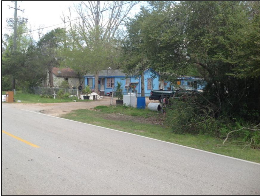
Figure 5: Single-family residence to the north.
