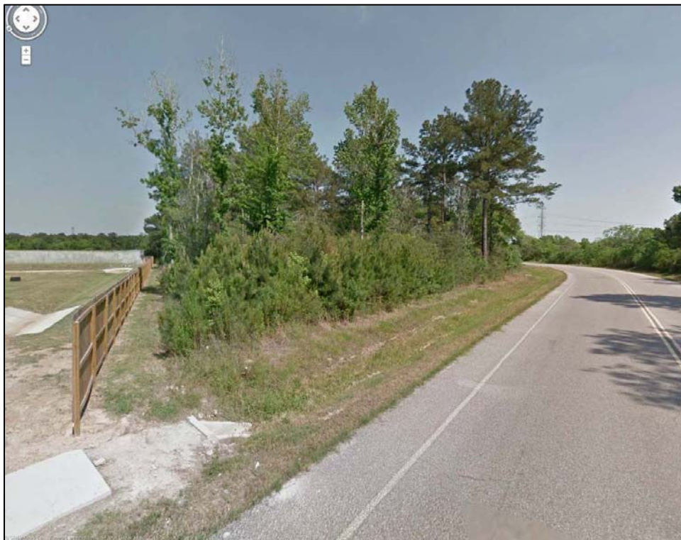
Figure 6: South of subject site.
