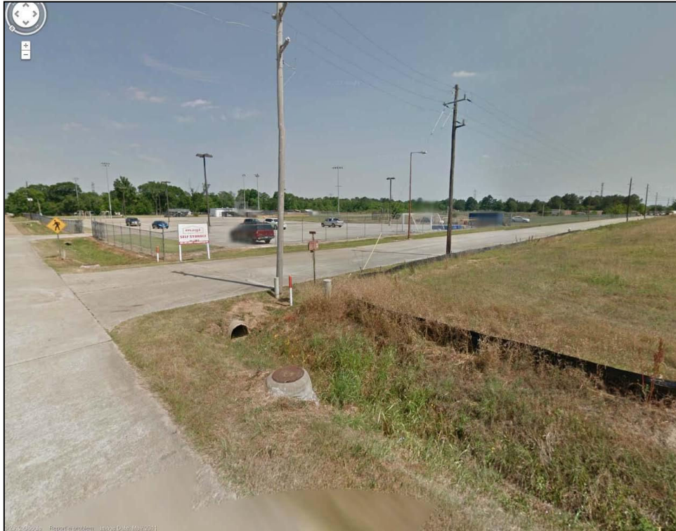
Figure 9: East of subject site.
