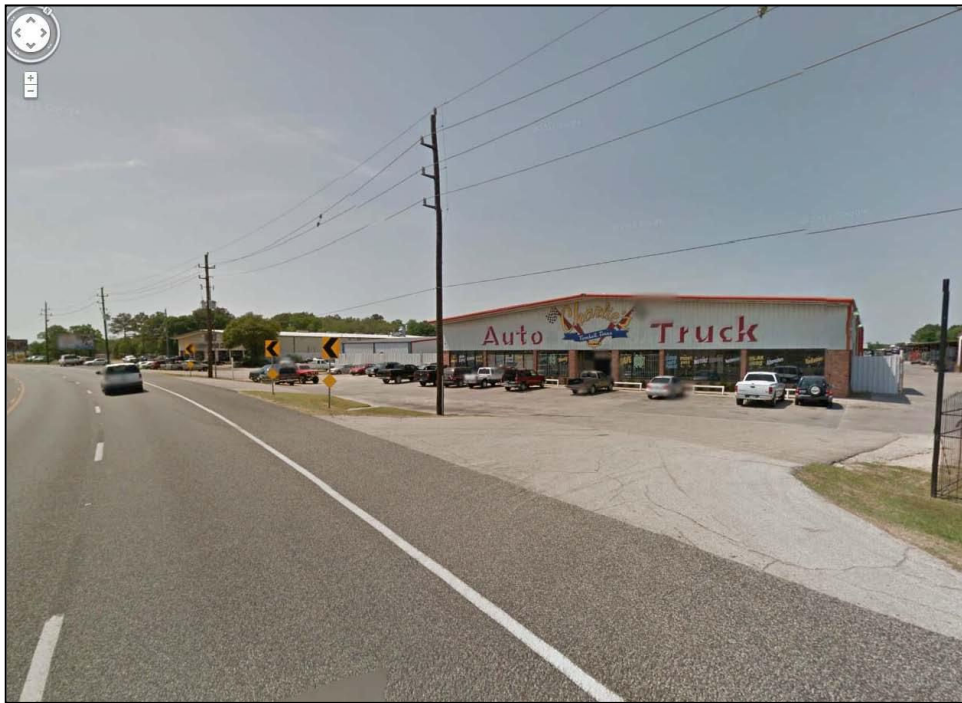
Figure 8: East of subject site.
