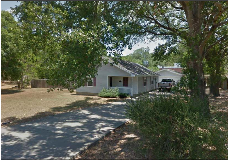
Figure 3: Single-family residence to the south. Source: maps.google.com
