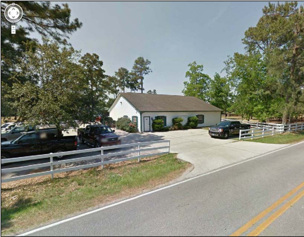
Figure 5: Contractor's office to the west. Source: maps.google.com
