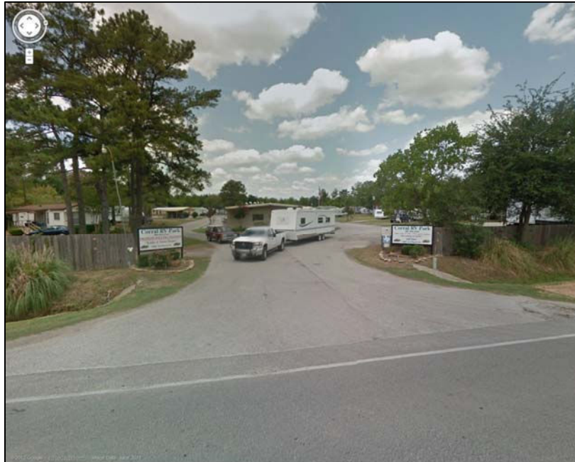
Figure 1: Subject site. Source: maps.google.com
