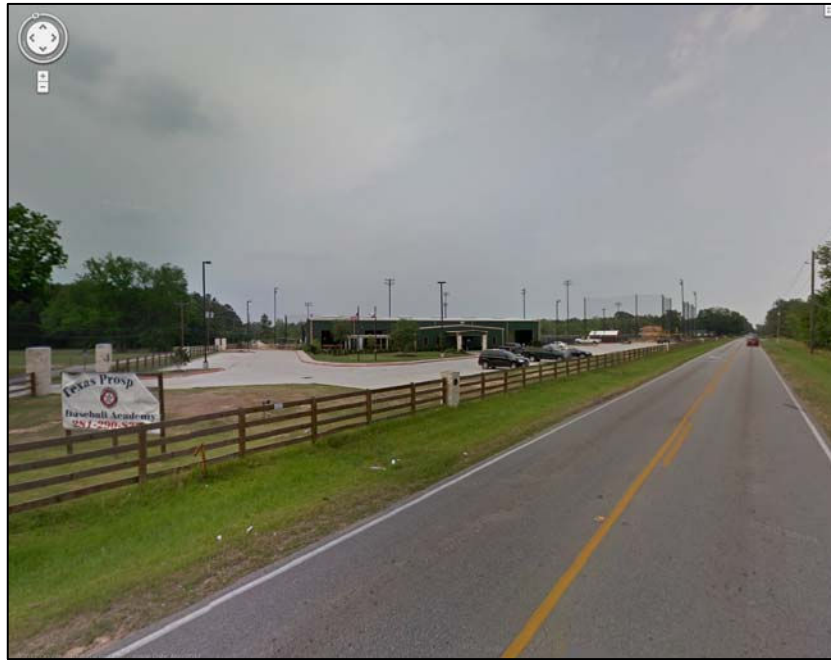
Figure 1: Subject site. Source: maps.google.com
