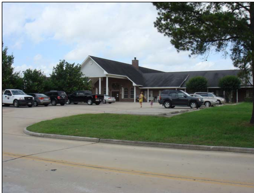
Figure 4: Assisted living facility to the west.
