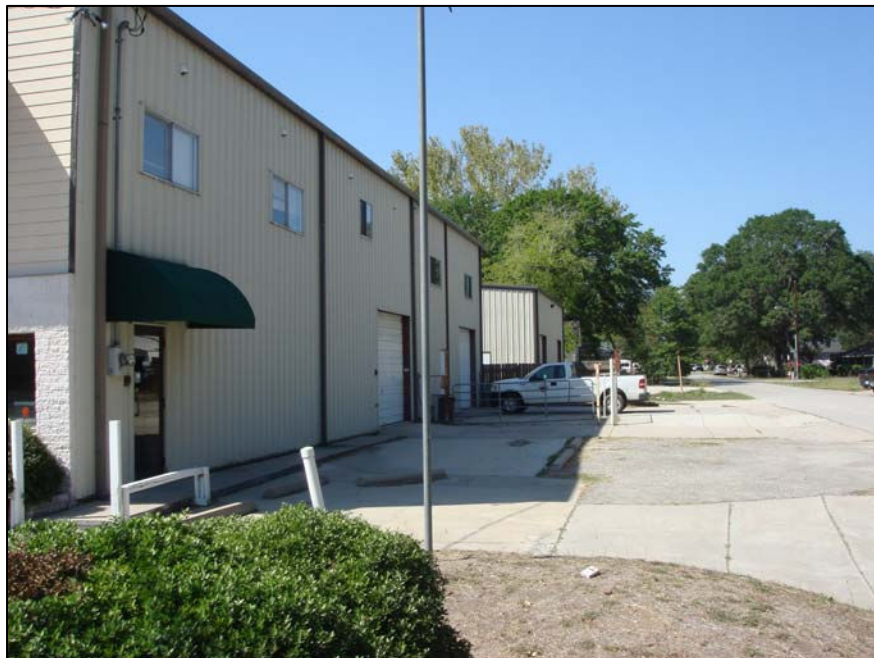
Figure 2: Easterly side of subject site.
