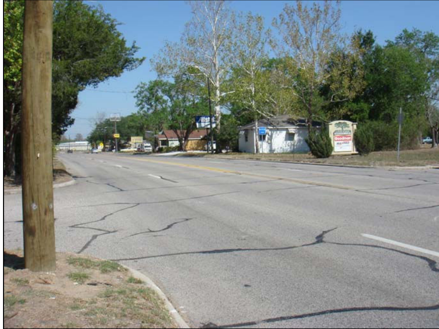
Figure 7: East of subject site.
