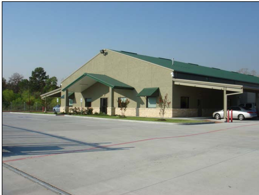
Figure 8: Creacom facility east of the subject site.
