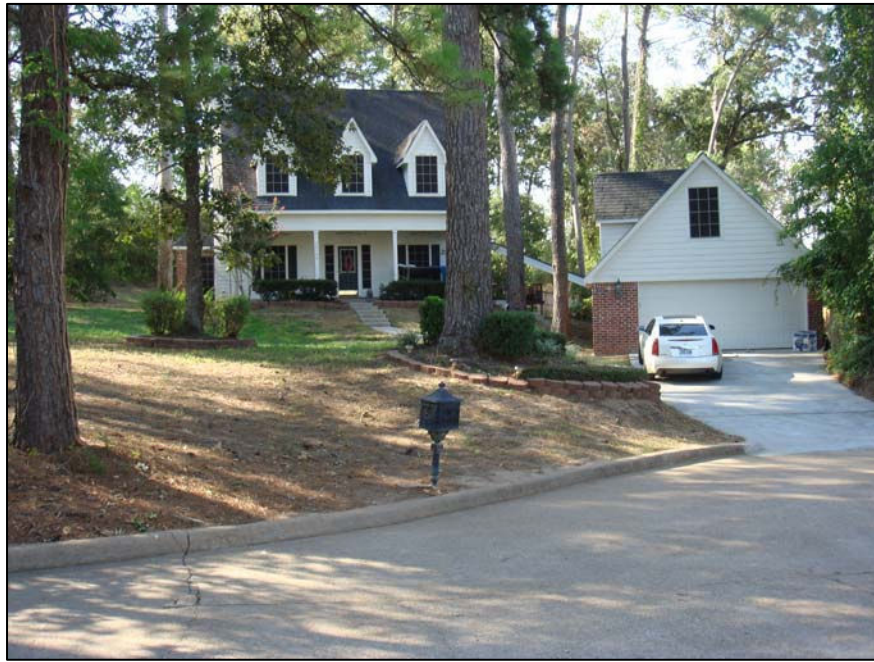
Figure 5: Single-family residence within Tomball Hills Subdivision to the east of subject site.
