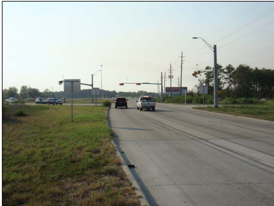
Figure 2: Southeasterly view down S.H. 249 Expressway. Subject site on right.
