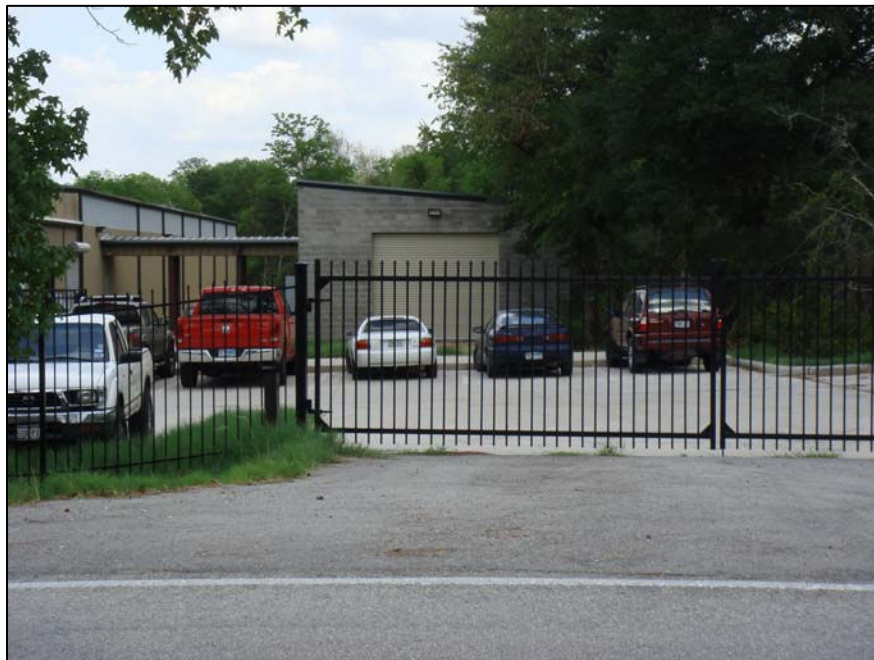
Figure 2: Easterly view of structure to be expanded.
