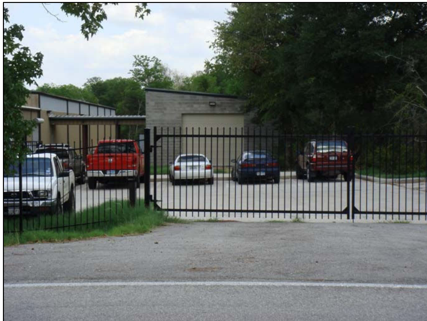
Figure 2: Easterly view of structure to be expanded.
