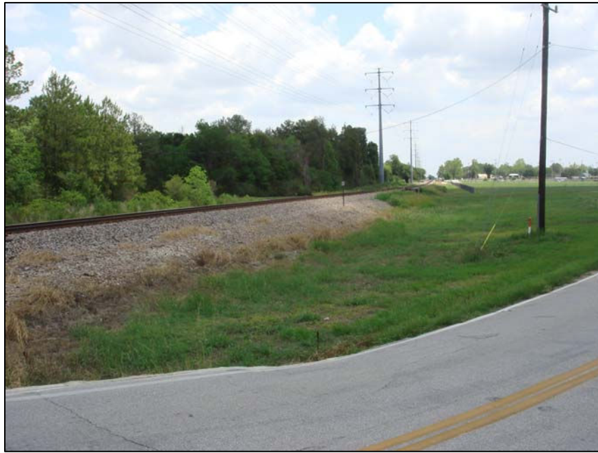
Figure 3: Southeasterly view. BNSF railway, City of Tomball property, and HCFCF drainage.
