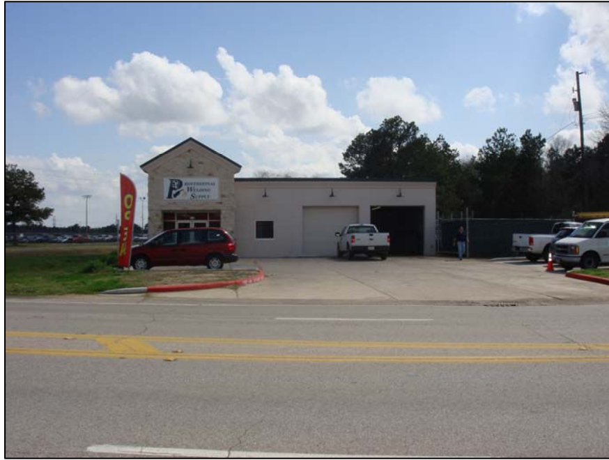
Figure 1: Southerly view of subject site.
