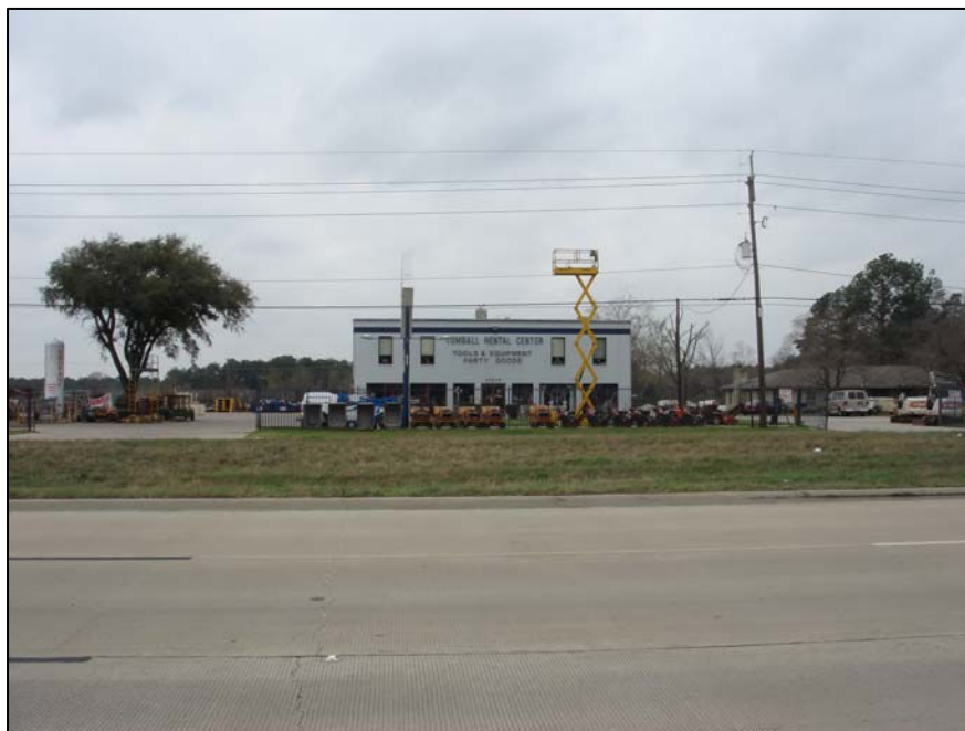
Figure 4: Tomball Rental Center to the south of subject site.
