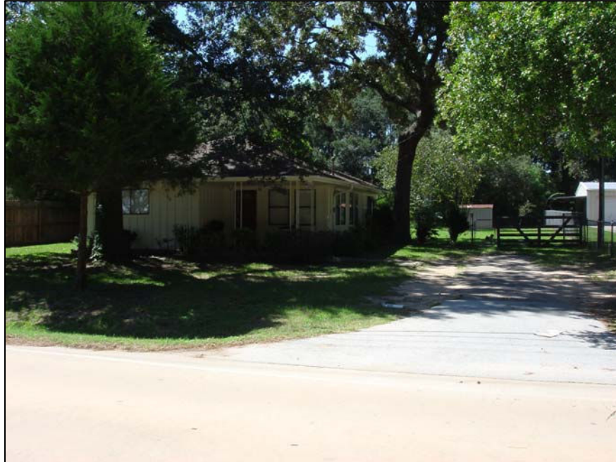
Figure 1: Westerly view of subject site.
